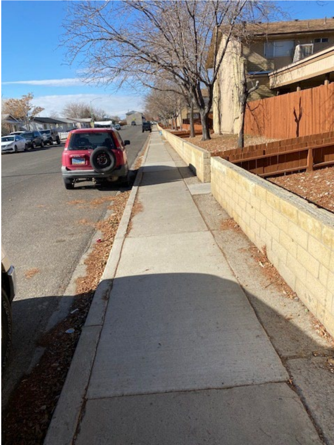
Repaired Sidewalk Sections
